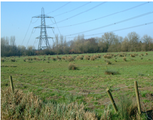
Overhead wires and pylons
