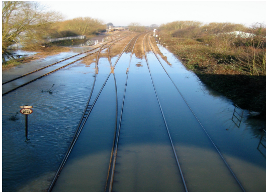
Flooded railway line in 2003
